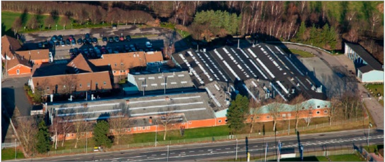
10,450 m 2 factory in Denmark, Headquarters of: scansteel foodtech A/S & Koncept Tech ApS
